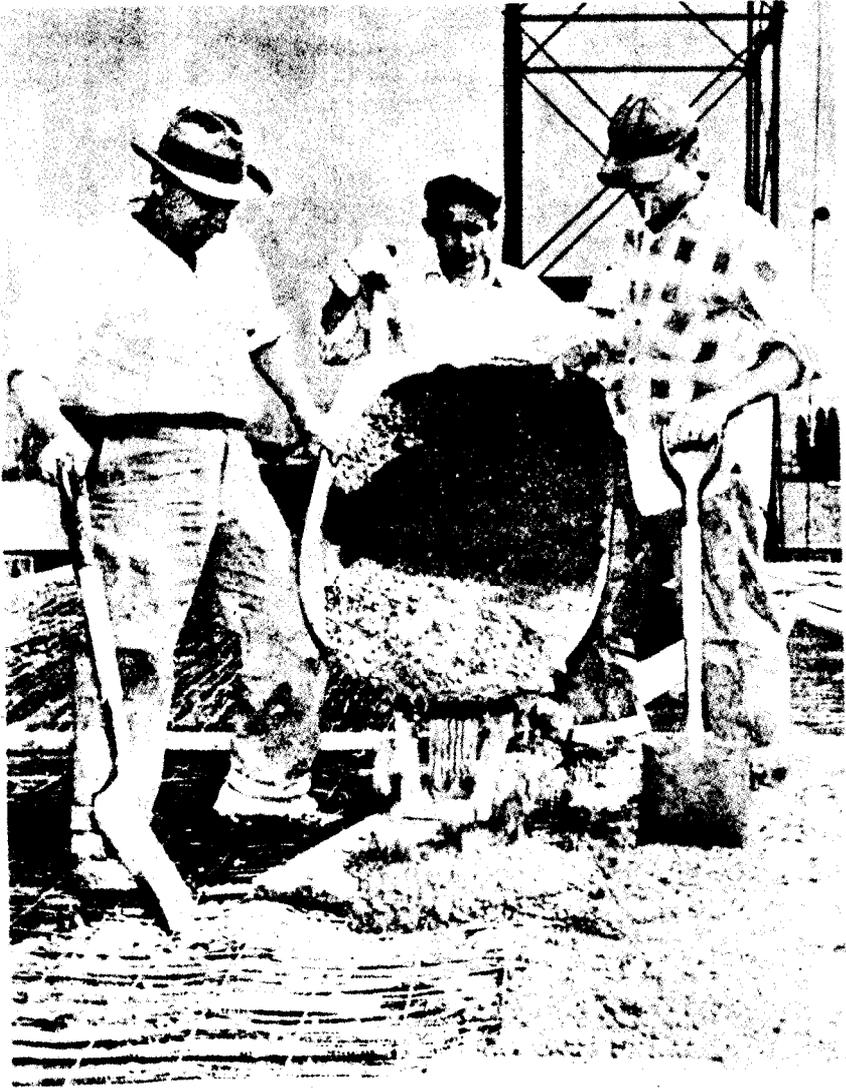
FIG. 31 PLACING CONCRETE FLOOR SLAB ABOVE OPEN WEB JOISTS
